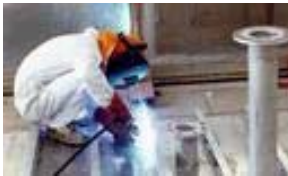
After applying C5, falling spatter is simply brushed away.
