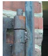
Repair damaged galvanized surfaces
